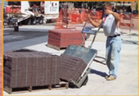
When tipping the PAVERCART back loaded with a band of pavers, grab the very top of the handles for improved leverage.
