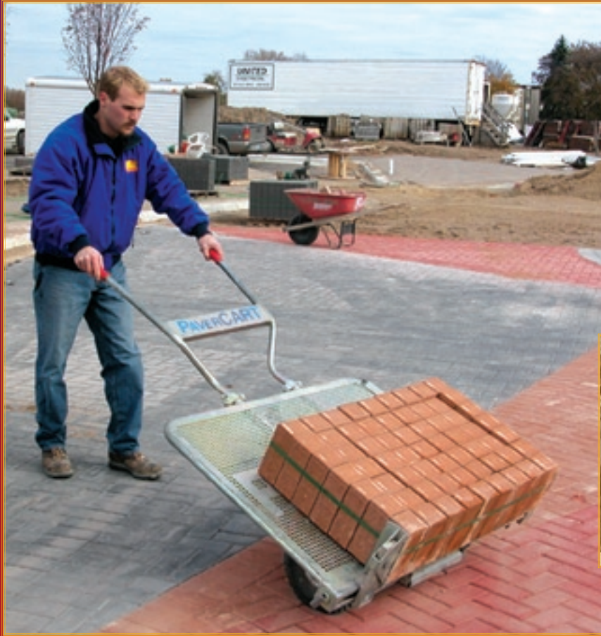
When tipping the PAVERCART back loaded with a band of pavers, grab the very top of the handles for improved leverage.
