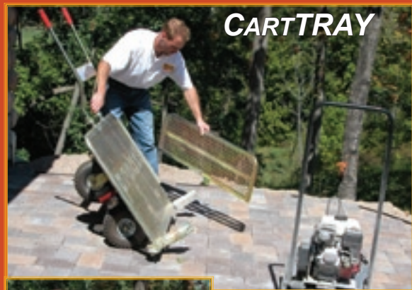
When tipping the PAVERCART back loaded with a band of pavers, grab the very top of the handles for improved leverage.
