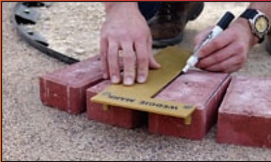
Line up the inside of the "L" with the first corner and mark; then move to the other corner and mark. Next, place the Wedgie Mark on the top of the paver to be marked. There are 2 pins that are attached to the bottom; these go against the sides of the pavers on the outside of the radius.
