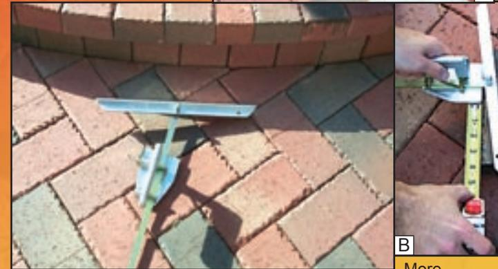
**A.** Set PAVERSCRIBE on Bond Line near center of where cut paver is to be set. Follow Step 2.
