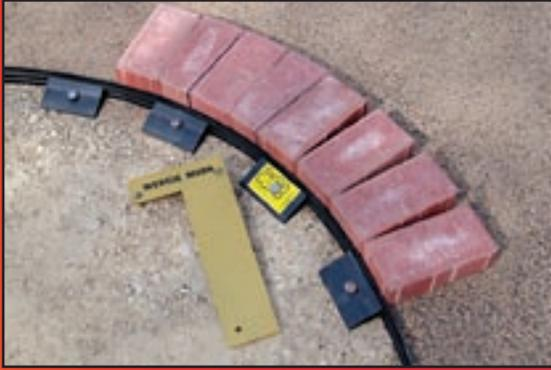
The Wedgie Mark is designed to mark for cutting the "soldier" course on both inside and outside curves. When cutting the "soldier" course pavers, mark both sides of every other paver. This reduces the amount of cutting compared to marking every paver and is more aesthetically pleasing compared to marking one side of every paver. First, lay in 3 full pavers and adjust so that the pavers are perpendicular to the edging and that the gaps are even on both sides of the paver to be marked.
