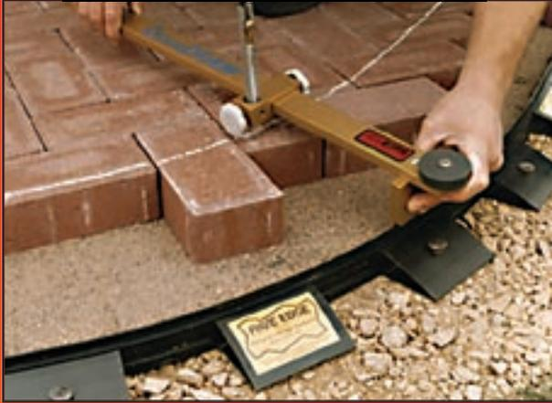
Marking pavers for a soldier course using a PAVE EDGE guide.
