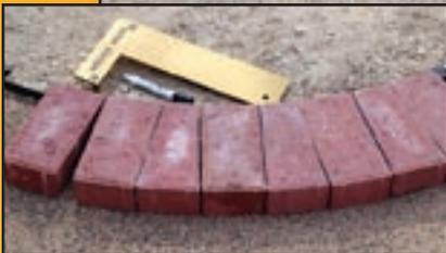
When both sides are marked, remove the paver and cut. If marked and cut properly, the cuts on both sides should end about a half inch from the end of the paver on the outside of the radius. This leaves a full paver width on all the paver on the
